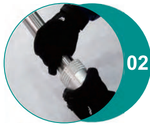
Deburr and chamfer the pipe end.
