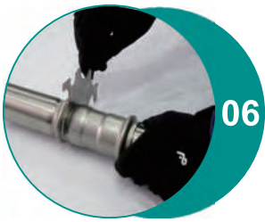
Use caliper to check and finish.
