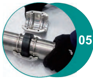
Position the clamp over the sealing element, make sure lugs are in the groove.
