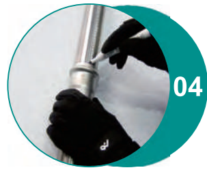
Mark the pipe with a marker pen.
