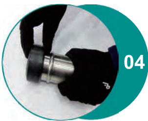
Insert pipes to the seal 2-3cm for both side.
